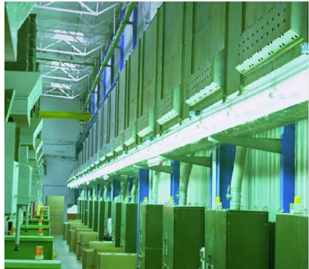
Air diffusers type LTB directly connected to the supply air duct, with lateral air injection.
