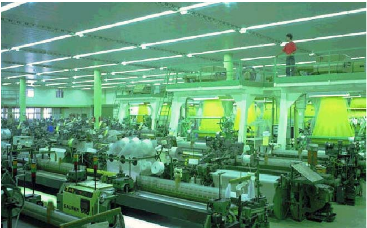
Air diffusers type LTB installed below the dropped ceiling with the supply air ducts above
